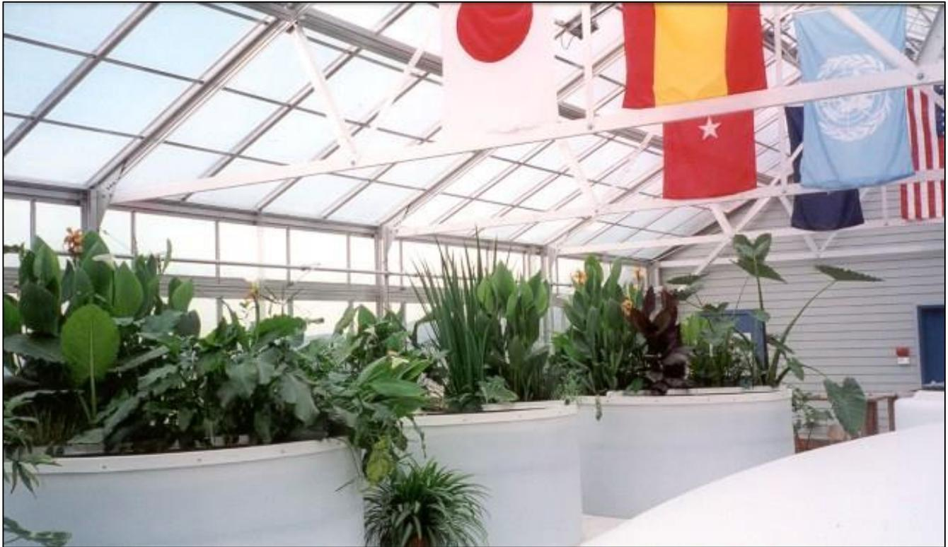
*Solar aquatic tanks treat effluent from Darrow's campus inside the greenhouse*
