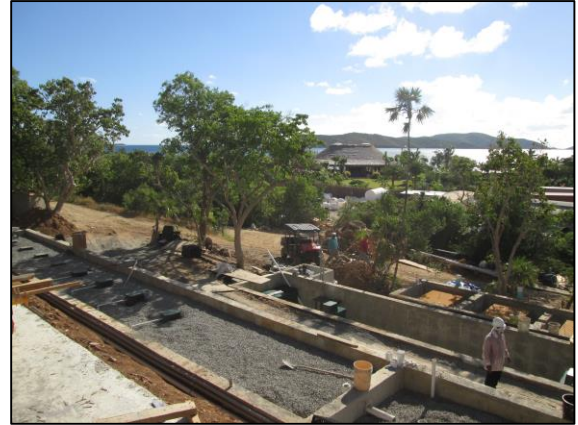
Wetland cells under construction
