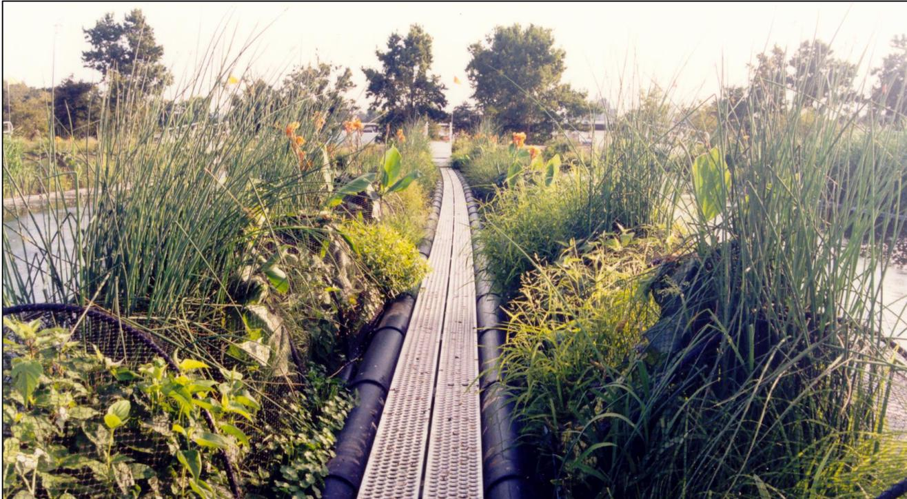
*One of the twelve Restorers installed at a chicken-processing waste lagoon*
