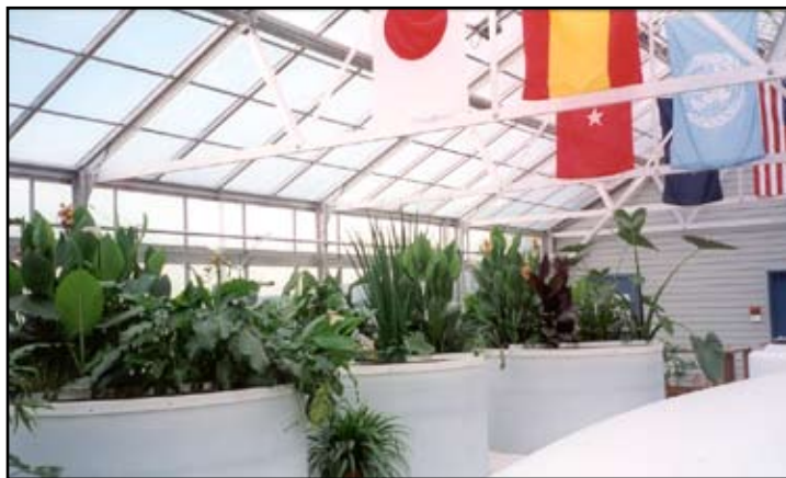
Lush vegetation of the five open aerobic aquatic cells enclosed in a vented greenhouse
